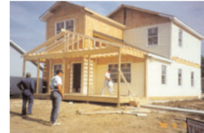
Site-built elements are the responsibility of the developer’s contractor (courtesy, MHI).
