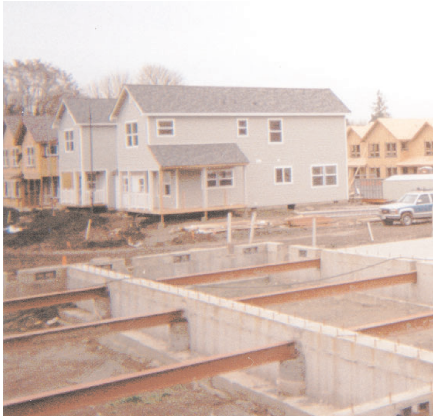
Noji Gardens manufactured homes are set on permanent foundations (courtesy, SWA).
