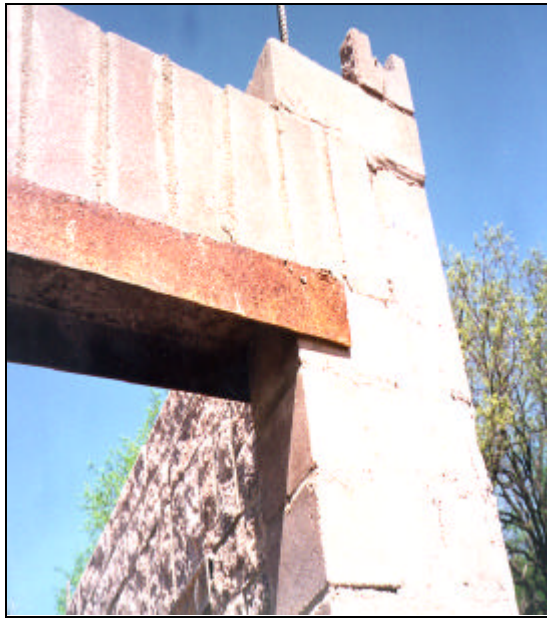
Photos 7a and 7b. Reinforced CMU Lintel at Minnesota Site (with and without temporary steel lintel).
