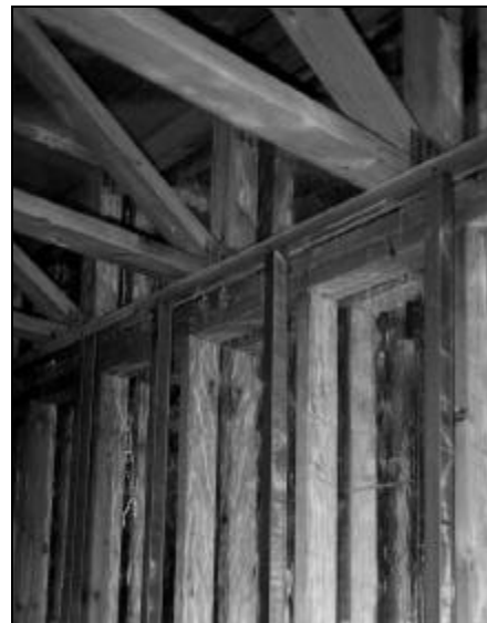
Photo 9 Floor Deck Connection at Minnesota Site
