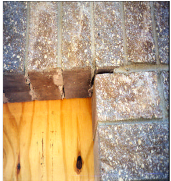
Photos 7a and 7b. Reinforced CMU Lintel at Minnesota Site (with and without temporary steel lintel).
