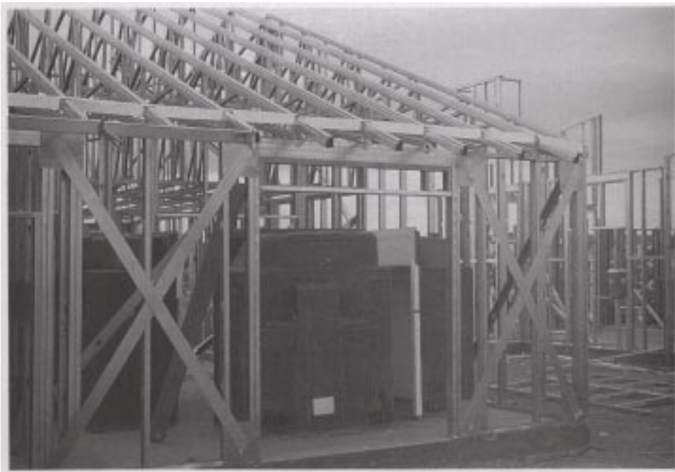
Photo 11. "IN-LINE" FRAMING TECHNIQUE
