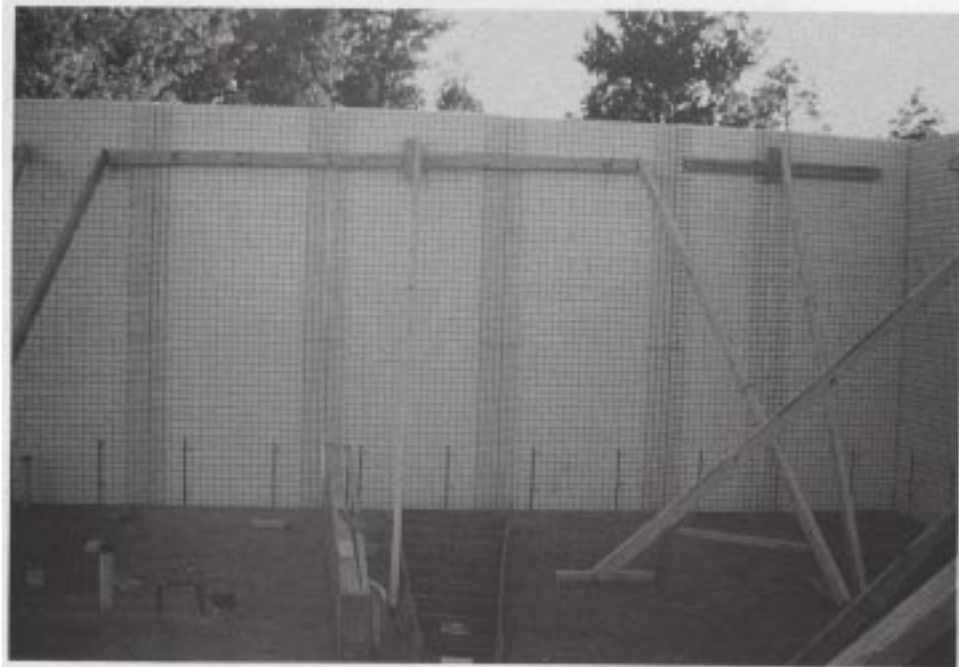
Photo 17. WWSP WALL BRACING
