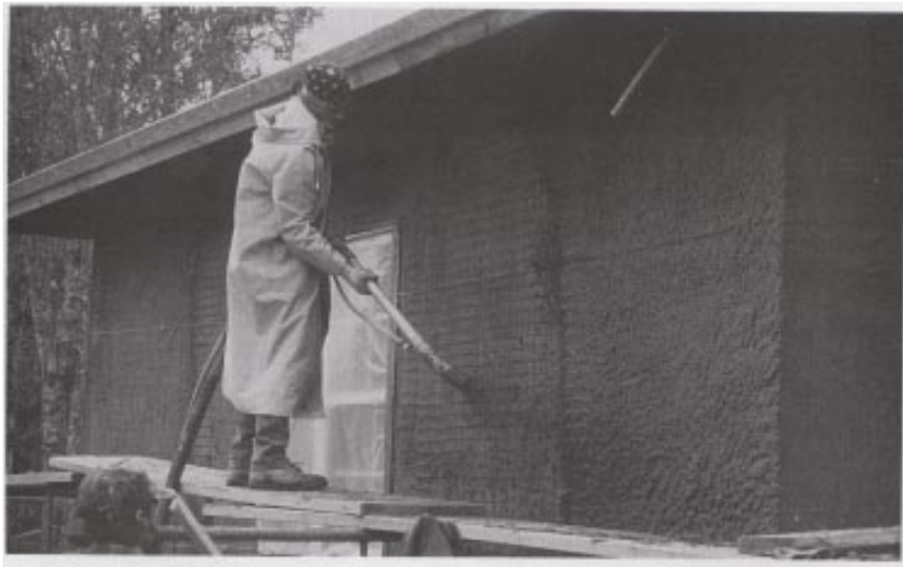
Photo 21. SHOTCRETE APPLICATION: FINISH COAT
