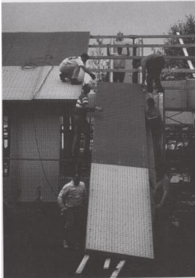
Photo 20. WWSP ROOF PANEL INSTALLATION
