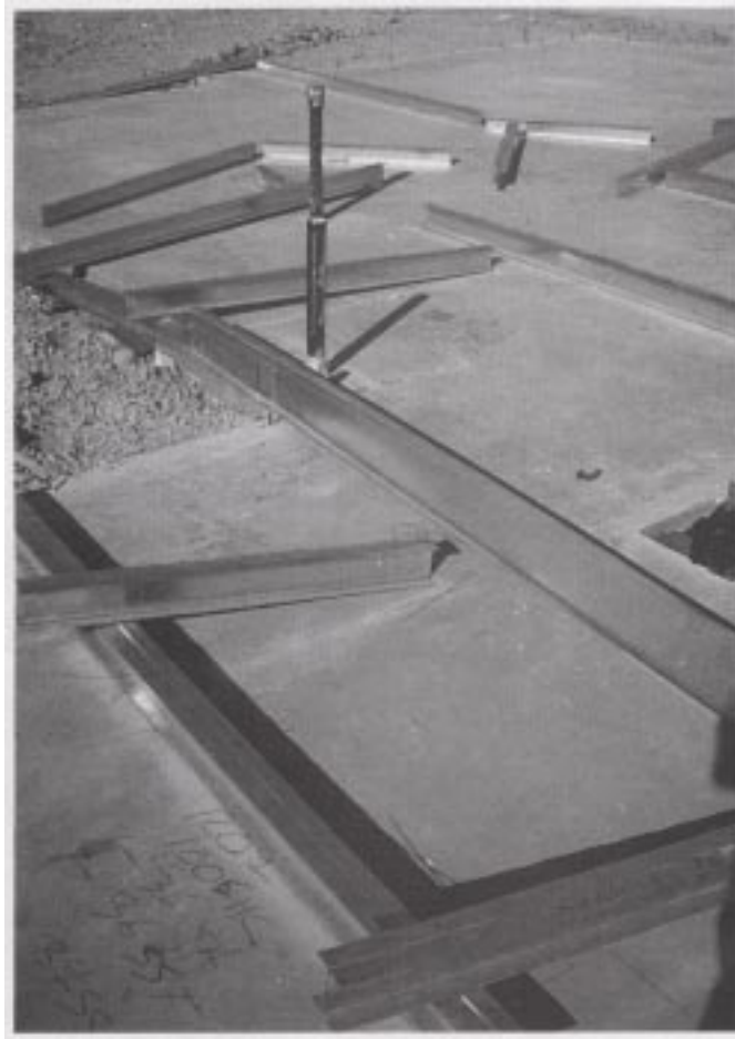
Photo 8. LIGHT-GAUGE STEEL LAYOUT OF TOP AND BOTTOM TRACK
