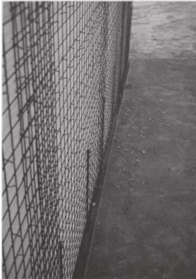
Photo 16. WWSPs TIED TO REBAR
