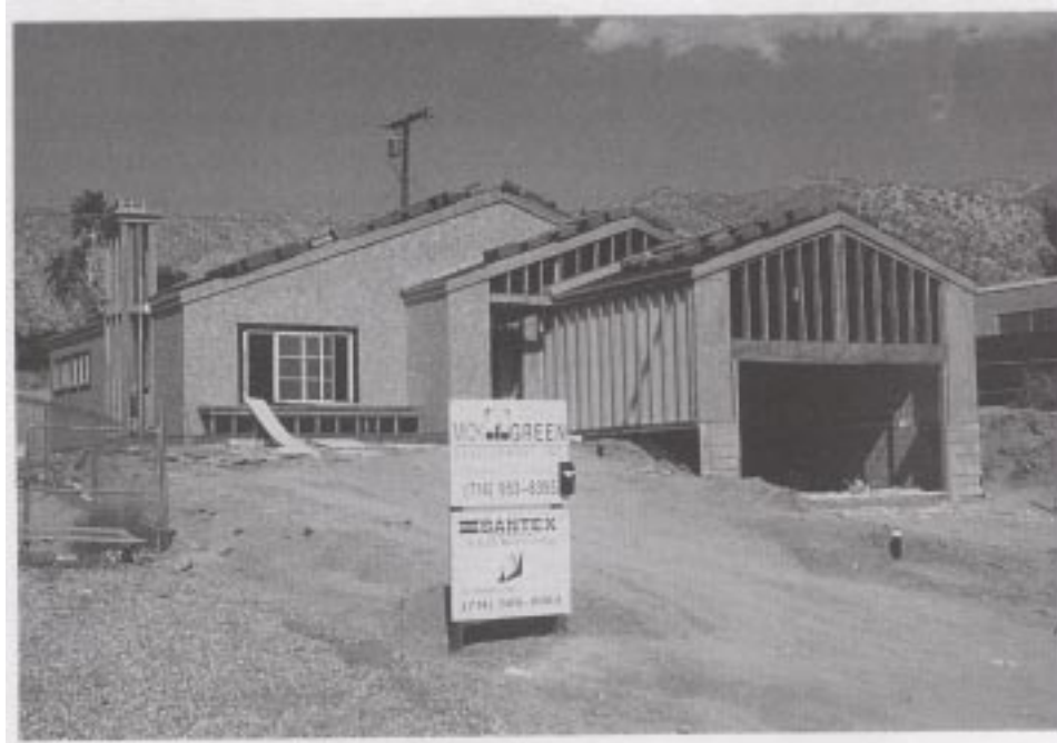
Photo 2. FOAM-CORE PANEL DEMONSTRATION HOME
