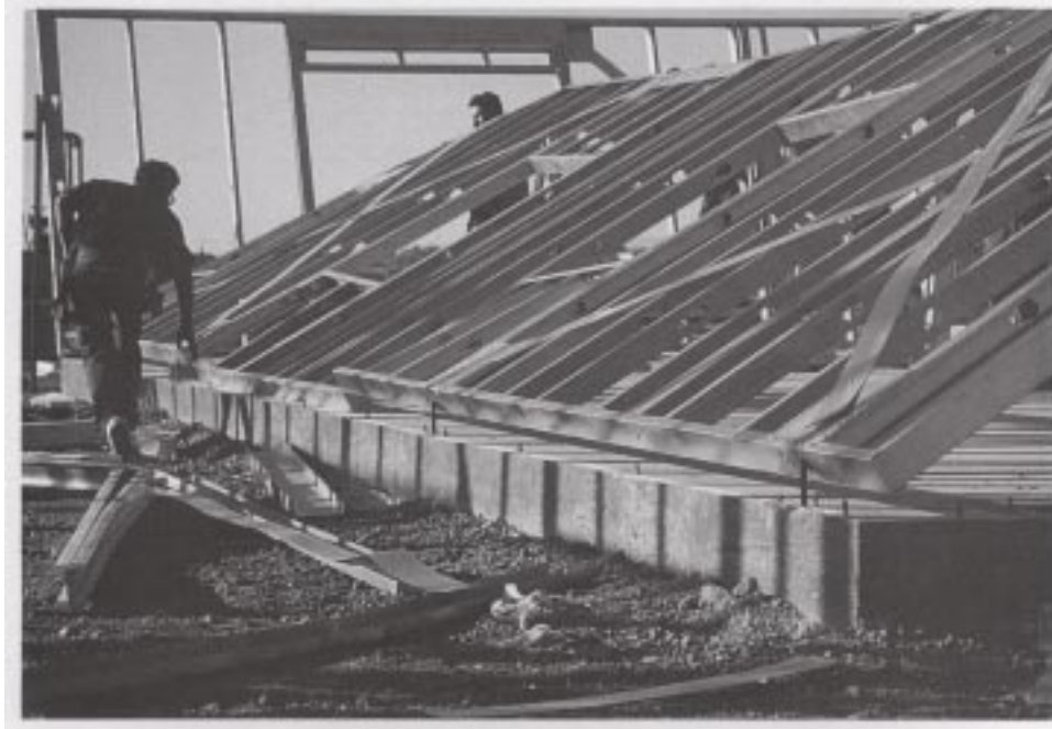
Photo 9. LIGHT-GAUGE STEEL WALLS BRACED IN POSITION
