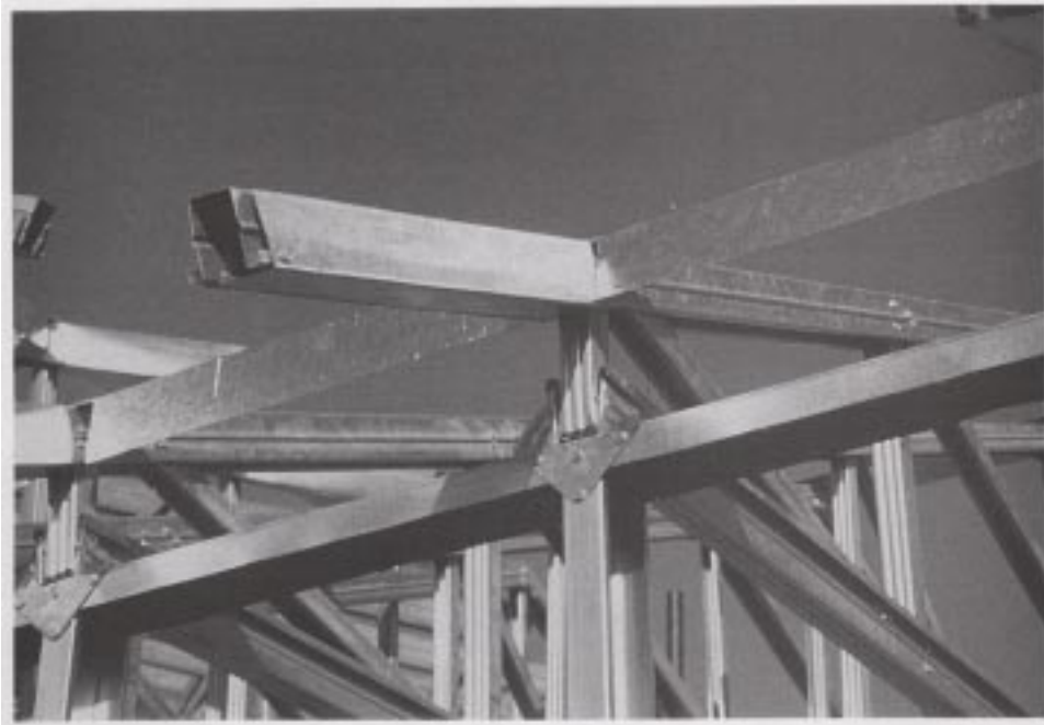
Photo 10. LIGHT-GAUGE STEEL SHEAR WALLS
