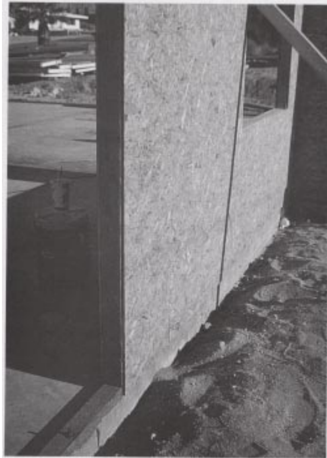
Photo 3. FOAM-CORE PANEL FASTENED TO SILL PLATE
