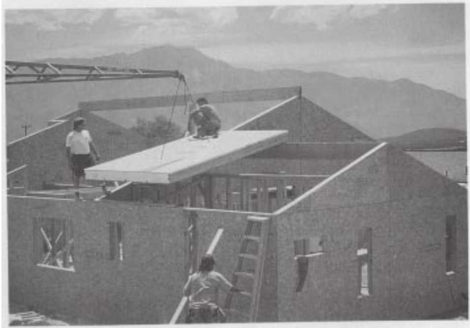
Photo 6. FOAM-CORE ROOF PANELS BEING SET IN POSITION
