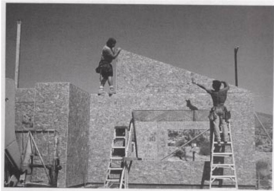
Photo 5. FOAM-CORE PANEL GABLE-END WALLS
