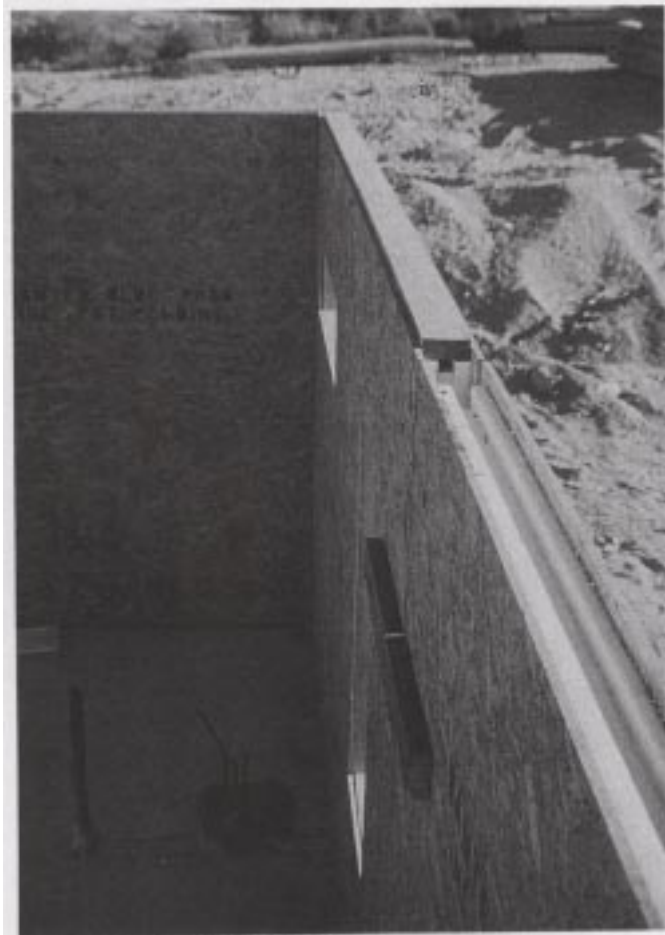
Photo 4. TOP OF FOAM-CORE PANEL FITTED WITH A TOP PLATE
