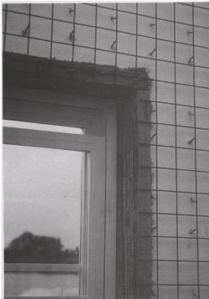
Photo 18. WWSP WINDOW FRAMING
